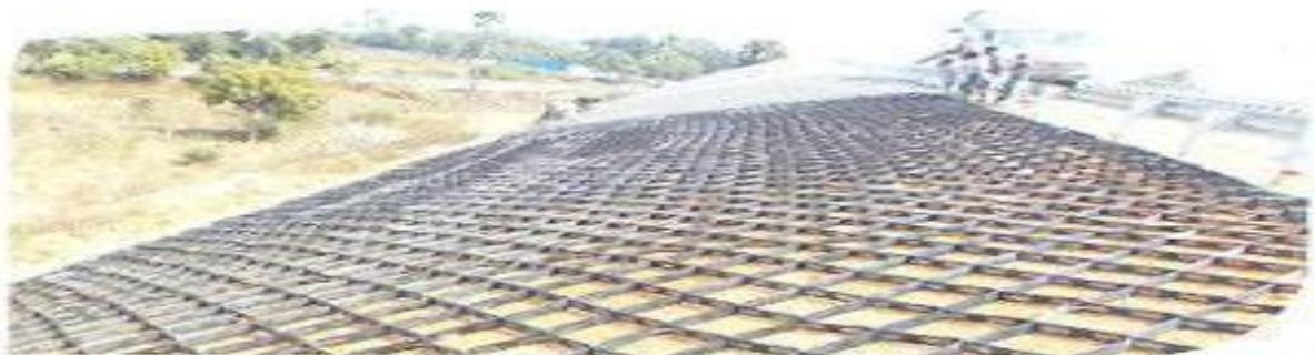
Embankment protection on national highway using geocell (STRATA)
